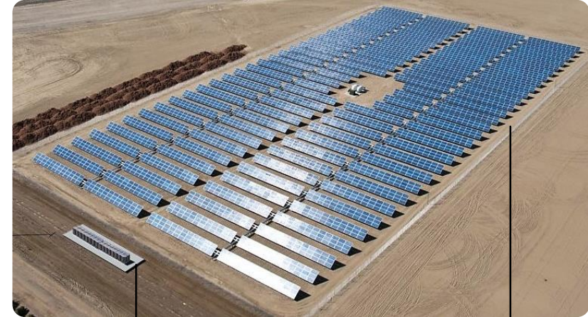
1 MW Solar PV Facility
